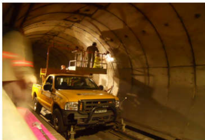
Figure 2. Installing the measuring section for tunnel monitoring
