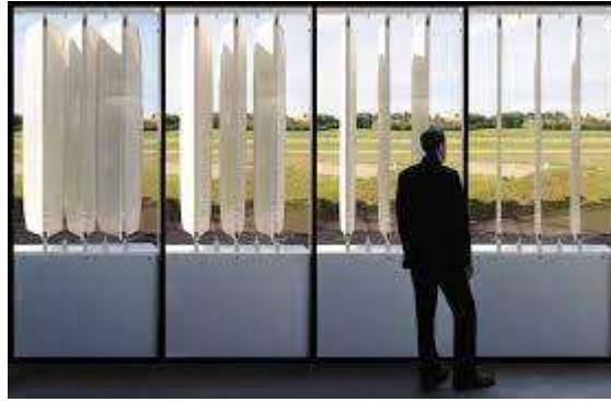
Figure 2 – The facade shading system based on the Flectofin produced in collaboration with the industrial partner Clauss Markisen [3].
