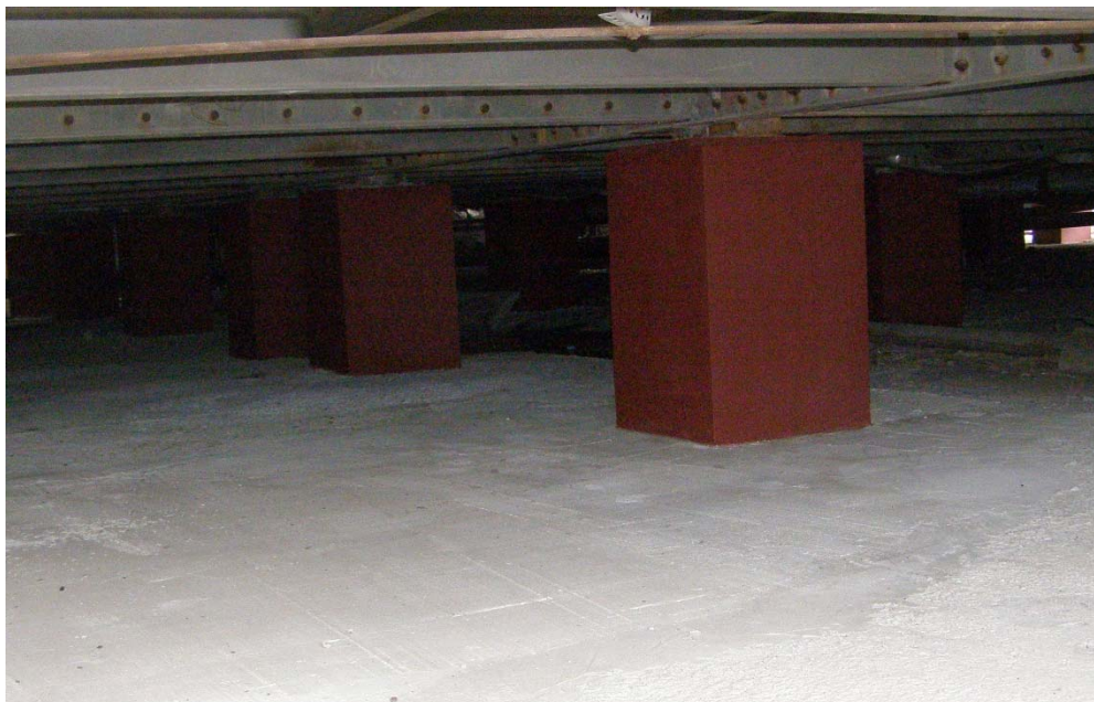
Figure 3 –The finished construction of foundation reinforcement.
