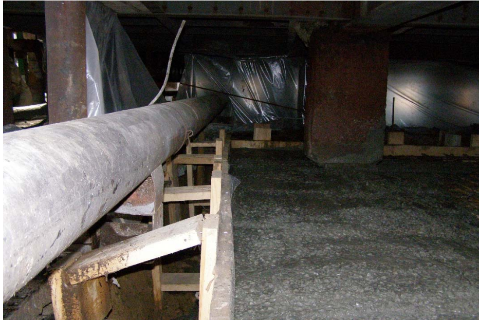
Figure 2 – The stage of concreting the foundation slab is strengthened without the use of vibration.
