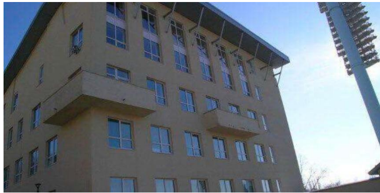
Рис. 3 – Lucky.Net Telecom Office
